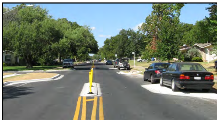
Curb extensions, lane divider, and speed tables on Rockwood. Photo by Daniel Barrera
